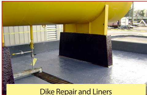
Dike Repair and Liners
