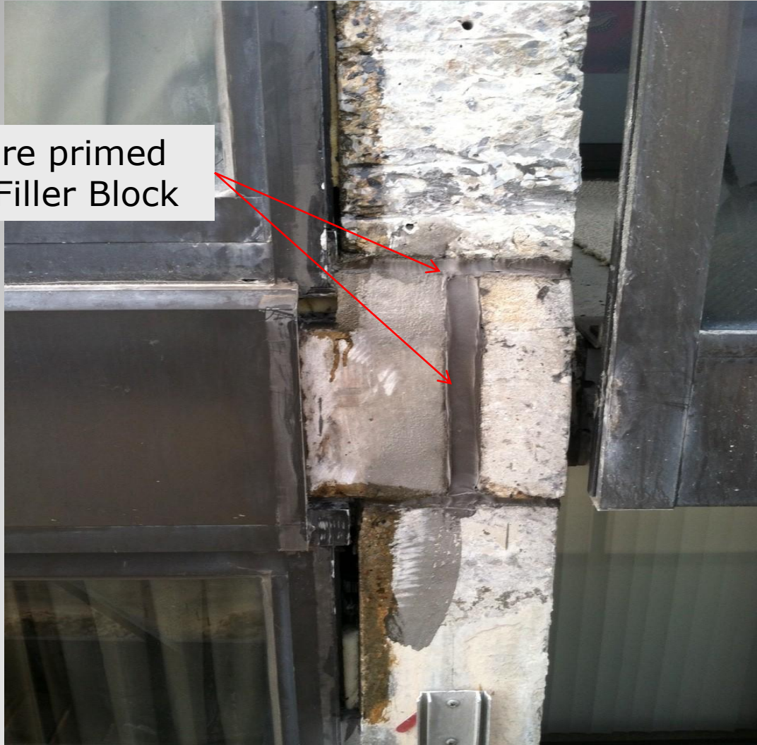
Golden Sands Hollow Core and Prestressed Beam/Column Construction
